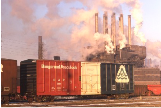
Rouge Power Plant
